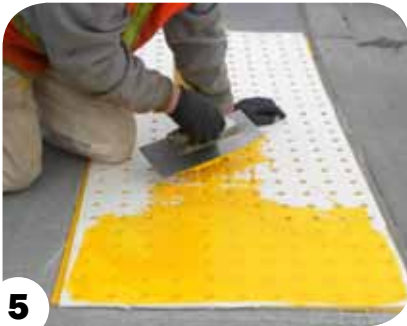
Apply liquid plastic dome material
