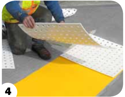
Apply dome template mats to SkidGuard
