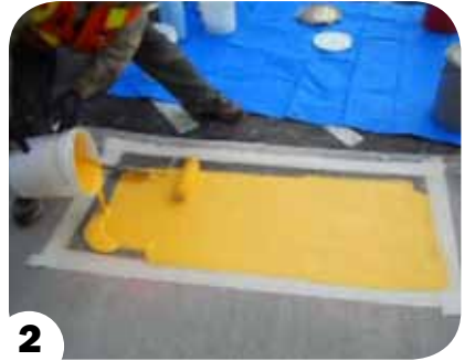
Apply liquid plastic SkidGuard
