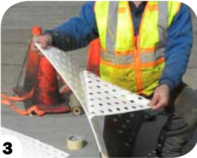
Peel wax paper off the adhesive backed template.
