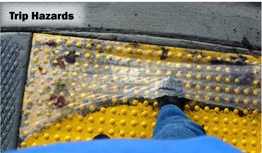
Solar/UV Deterioration
